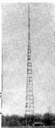
Truscon Type H-30 Self-Supporting Tower, operated by WEXL-FM, Detroit, Mich., supports an 8-bay General Electric FM antenna and rises to an overall height of 425 feet.
