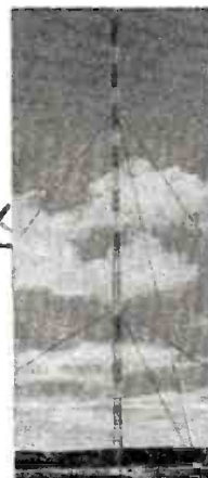
Truscon Guyed Radio Tower, WKY, Oklahoma City, Okla., is 956 feet high to top of FM antenna.
