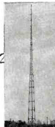
WUSJ-FM, Lockport, N. Y. Truscon Self-Supporting Tower, 135 feet high and supporting a GE 4-bay FM antenna 42 feet high. Overall height 177 feet.
