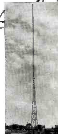
This 240 foot Truscon Tower, operated by WTCH, Shawano, Wisconsin, has 52x48 Truscon Ground Screen to assure an excellent signal.
